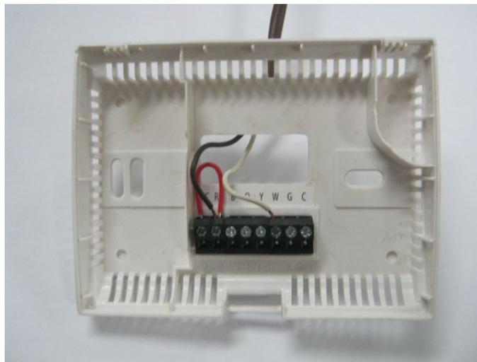
Connect one wire on "RH" and the other wire on "W". Red wire jumper can remain installed. For further information refer to the manufacturer's instructions.
