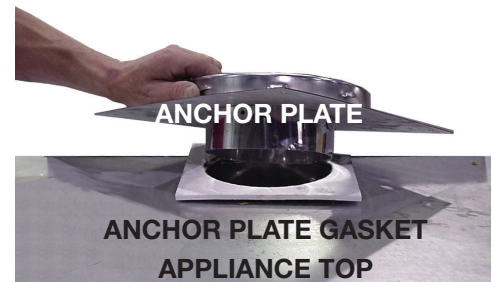
ANCHOR PLATE FOR A FACTORY BUILT CHIMNEY
