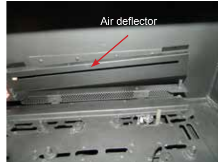
Install the rear air deflector to the back wall of the firebox using 2 existing lower 1/4" screws.
