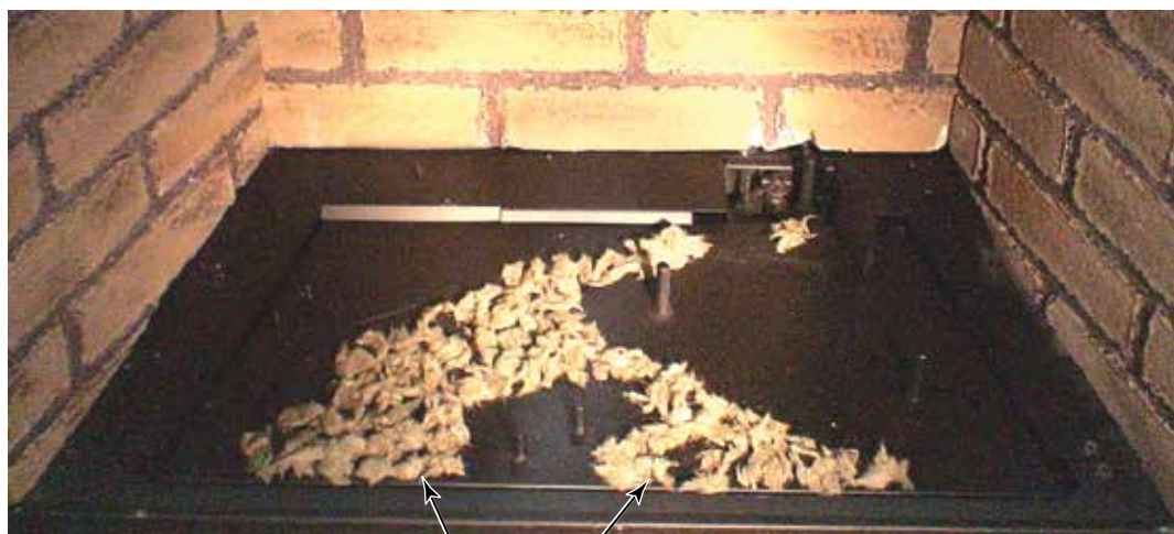
Figure 17b - Place Ember Material
