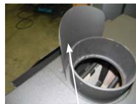
Installed Pipe Shield
