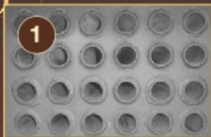
Heat exchanger with reverse return 2" diameter fire tubes.
