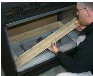
Remove the 2 Long Base Brick Panels
