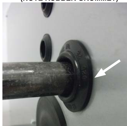
FIGURE 27 - FURNACE GAS PIPE CONNECTIONS (NOTE RUBBER GROMMET)
