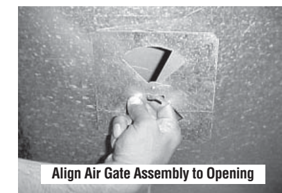
Figure 12 - Position Air Gate
