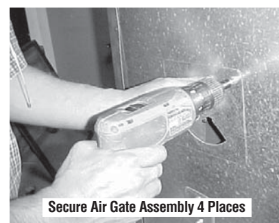
Figure 13 - Install Screws
