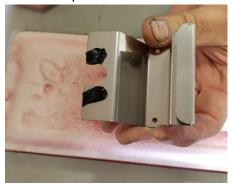
3. Slide clip into place on tile. See photos for proper placement.
