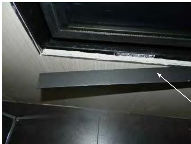
Figure 101: Top View - Sliding trim into place
