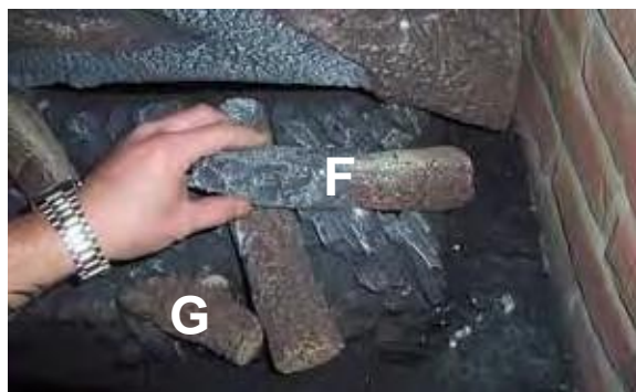
Figure 95: Log F and G position
