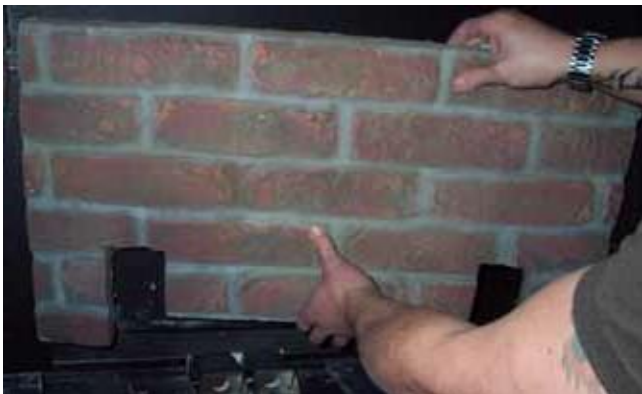
Figure 77: Lower Back Brick Panel
