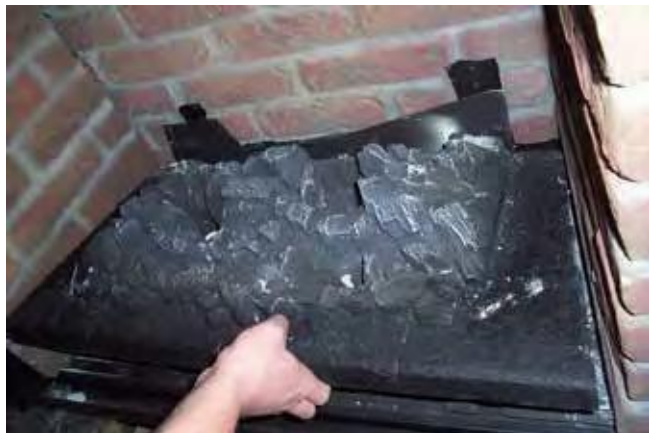
Figure 79: Burner Removal
