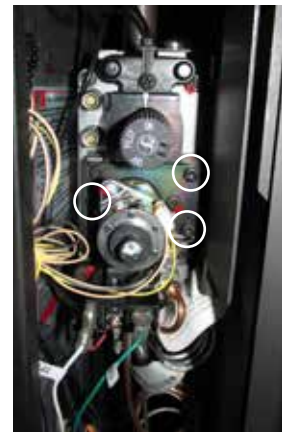
Remove NG Stepper motor and replace with LP Stepper motor
