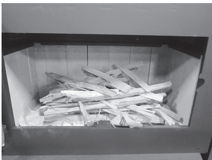
Figure 3.21 Placing Kindling
