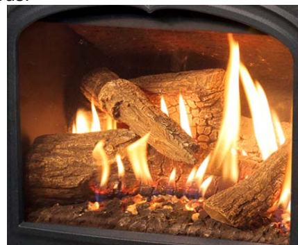
Figure 20: Apparence normale de la flamme
