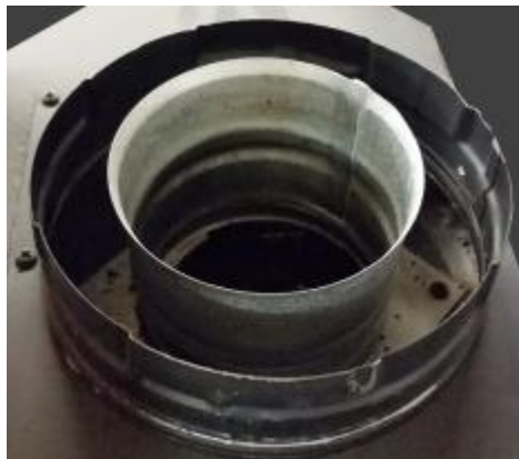
Vent Attachment Inspection – unbent and attached rings
