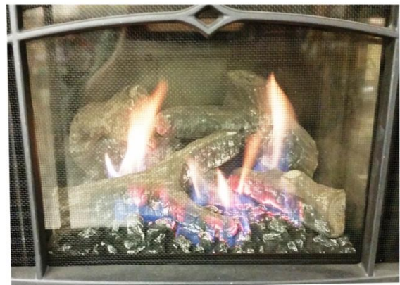
Figure 40 – Typical Burner Flame Appearance
