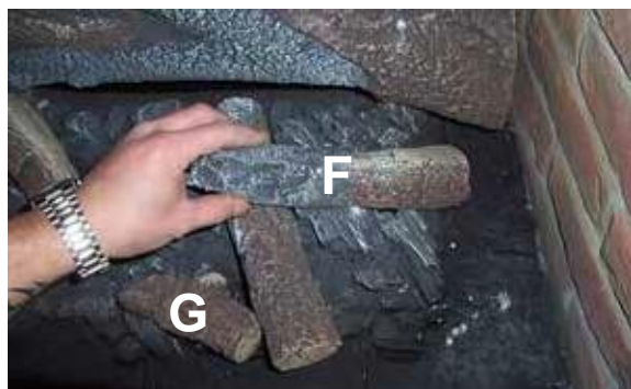
Figure 95: Log F and G position
