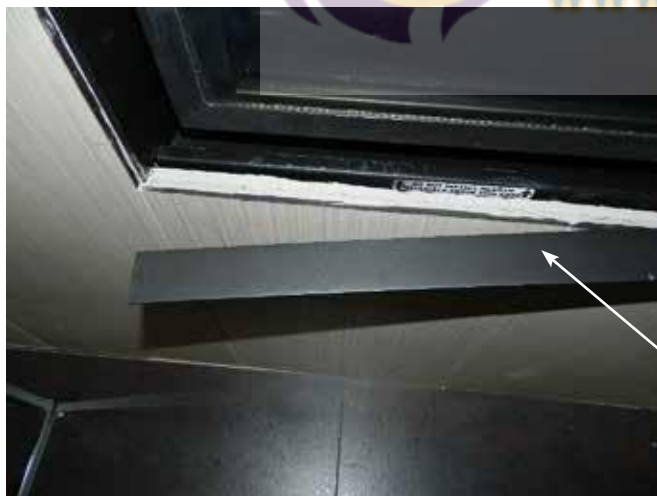
Figure 101: Top View - Sliding trim into place
