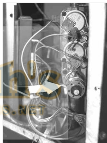
Figure 58: Modulator Screws.
