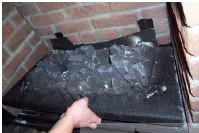
Figure 79: Burner Removal
