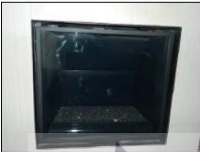
Figure 96: Glass Frame secured to the Unit
