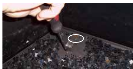
HZ33CE - install bracket, left side
