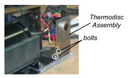
the fan motor, by detaching the phillips screw. Keep the screw to reattach the green ground wire on the other side.
