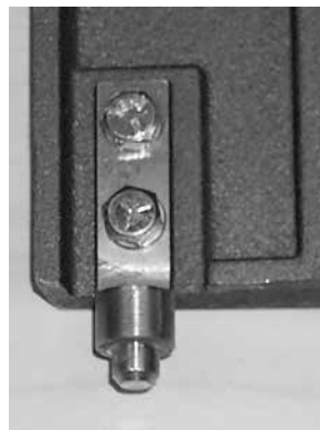
Bottom part of door fits into slot.
