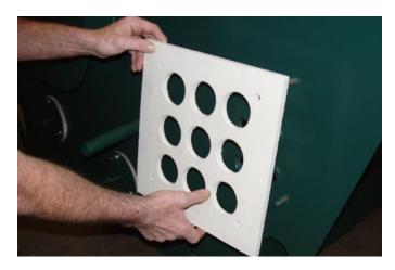
3) Align the junction box with the bolts and push against the insulation gasket.
