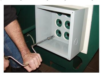
5) Affix the cover after leak testing and electrical installation.
