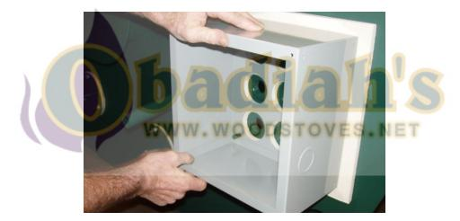
4) With the nuts provided, tighten the box against the gasket until the gasket compresses slightly.
