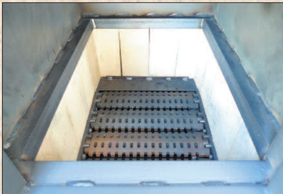
Inside Fire Box.
