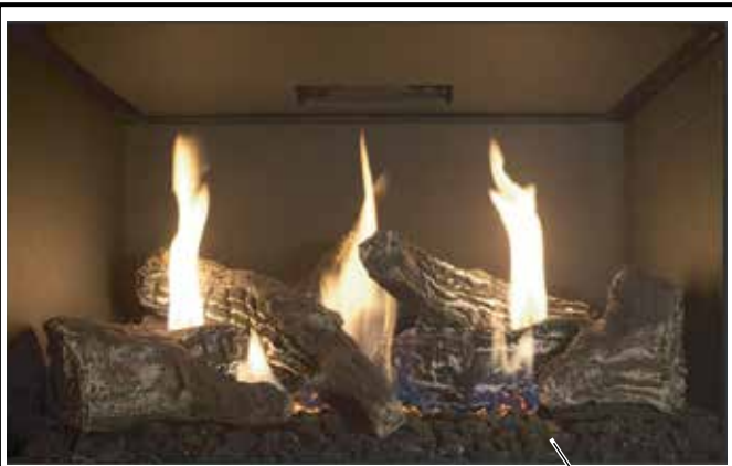
Figure 12 - Installing the volcanic stone
