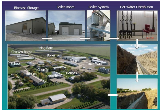
Figure 8-1: Diagram of Biomass District Heating System 29
