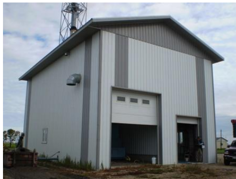
Figure 8-4: Biomass Heating System Building
