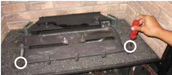
Diagram 1: Remove the left and right screws.
