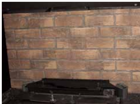
Back Panel Installed
