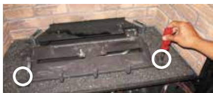
Diagram 1: Remove the left and right screws.
