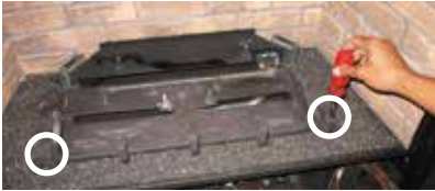
Diagram 1: Remove the left and right screws.
