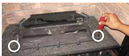
Diagram 1: Remove the left and right screws.
