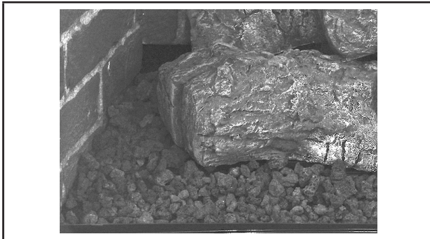
Figure 47: Installing the volcanic stone
