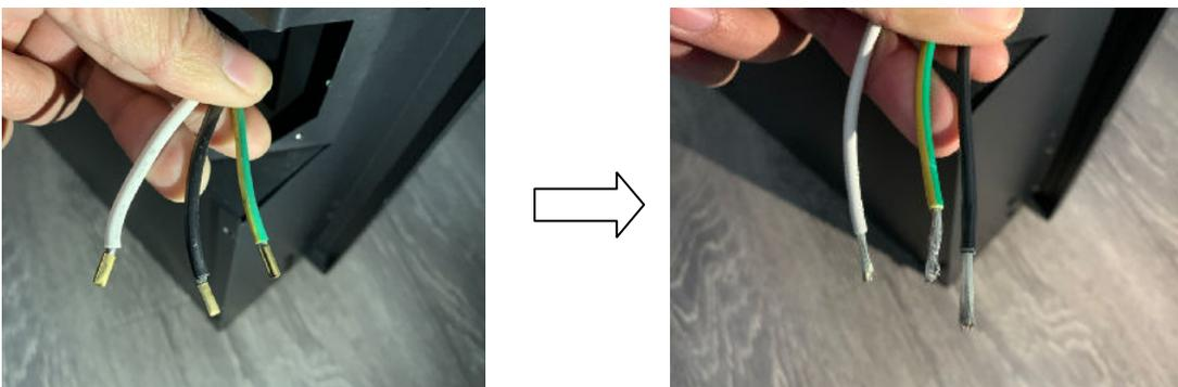
3. Connect the uncovered wiring with 14 A WG wiring (not provided with the appliance) by a wiring connecting cap which you can find in the manual bag. Please make sure the live wire goes into the “L”, the neutral wire into “N” and the ground wire into “G”.
