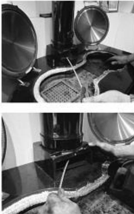
Remove the front of the flue connector box and insert the flue brush from left to right, angling the brush down at 45°. Once you find the flue way entrance push the brush down until it stops then gently but firmly pull back and forth 3 or 4 times then remove the brush. Dislodged soot will fall into the tray between the ovens.
