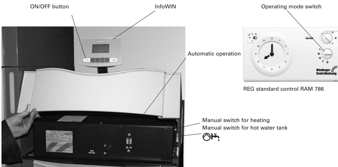
Fig. 106 BioWIN with REG standard control
