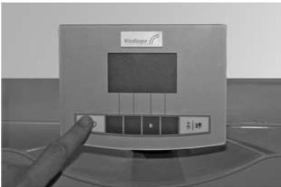
Fig. 111 Switching off BioWIN
