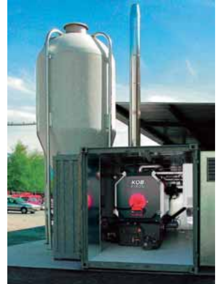
Portable boiler enclosure (pellet silo field supplied)
