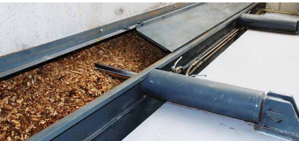
Walking floor installation
