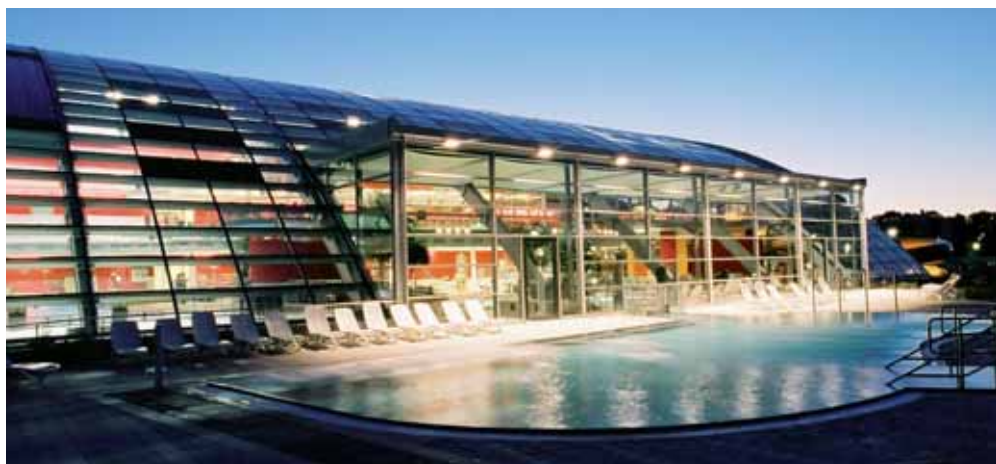
One of Germany's largest facilities powered by KÖB biomass heating technology. Recreational Pool and Spa. Kempten, Germany.
