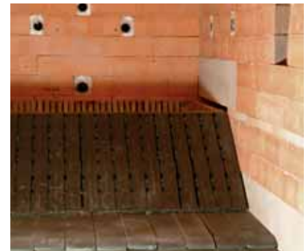
Firebrick-lined combustion chamber with external grate and moving annealing grate.
