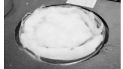
Step 3: Remove insulation from inside flue pipe.
