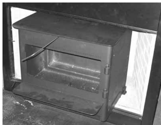
Schéma 5: Pull Rod In Place
