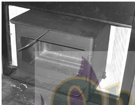
Diagram 5: Pull Rod In Place
