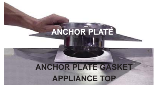
ANCHOR PLATE FOR A FACTORY BUILT CHIMNEY
