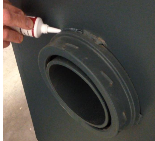
Step 2: apply silicone to welded seam between flue ring and tank head
