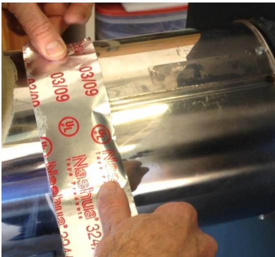
Step 5: Seal flue joints with aluminum tape or silicone (tape can be more easily removed)
