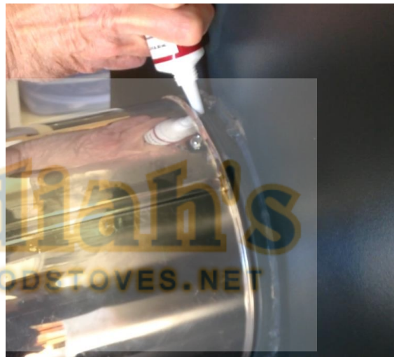
Step 4: Apply silicone to the seam between the flue and flue ring
