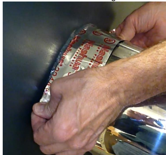
Step 5: Seal the flue joint to the flue ring.
