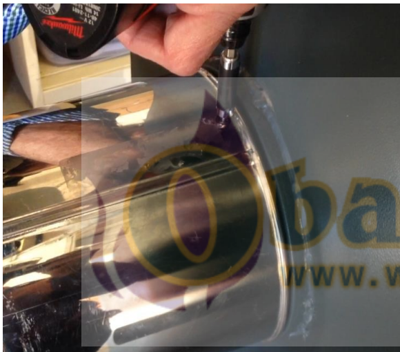
Step 3: Secure the flue to the flue ring and attach with sheet metal screws.
