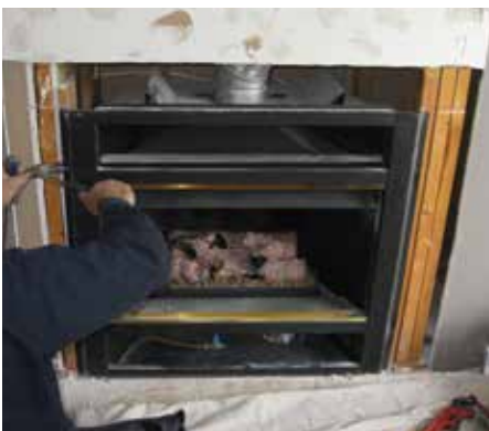
Remove unit from framing
