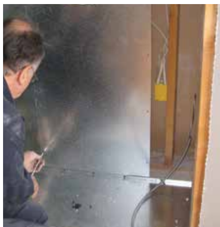
Fasten ZC box sections with provided screws.
