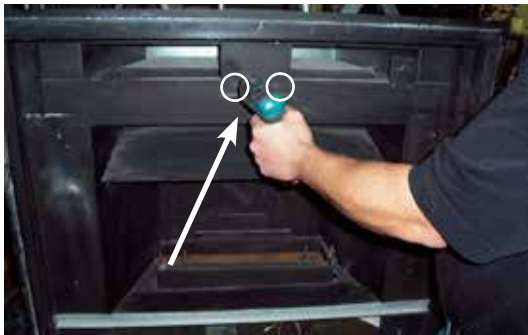
Remove 2 screws - remove Top Bracket
