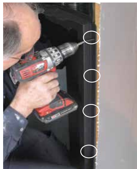
Use 4 screws on each side to secure surround and ZC box to studs.
