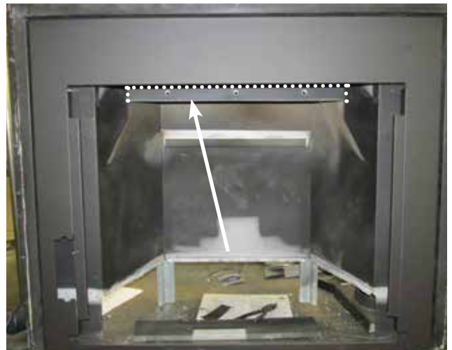
Cut out back cross bar
