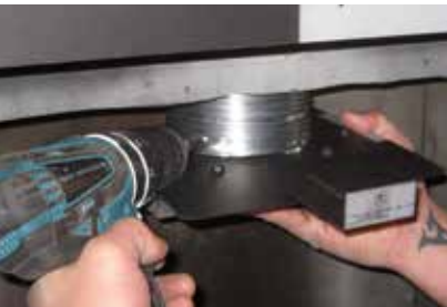
Secure vent slide plate to flex pipe with 4 screws
