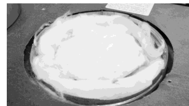
Step 3: Remove insulation from inside flue pipe.
