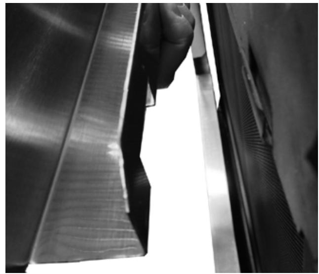
**Step 4a.** Slide the foot tabs of the facade base into the slots (see **Figure 41**) on both sides near the bottom of the fireplace opening.
