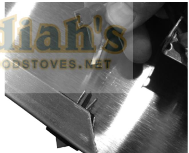
**NOTE:** Remove protective film from all stainless components before installation.
