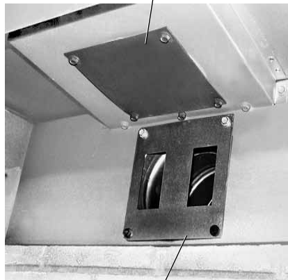
Rear Vent Restrictor Plate (shown installed over rear vent hole after Rear Solid Cover Plate was removed)
